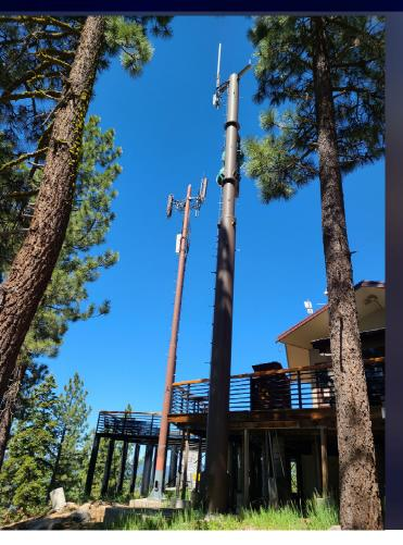
Snowflake lodge needs conduit installed from Equipment room (room next to ski patrol) over to the monopole. Current conduit is full of cable, with no ability to remove cables and install anything new.
